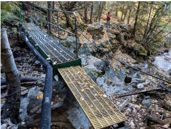
Photo 3. Fan apex below water system
