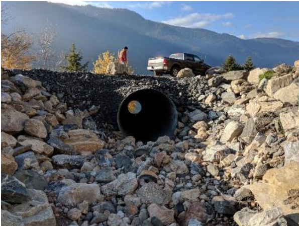
Photo 7. 2500mm diameter culvert at Broadwater Road
