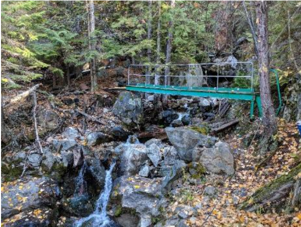
Photo 1. Water system access bridge
